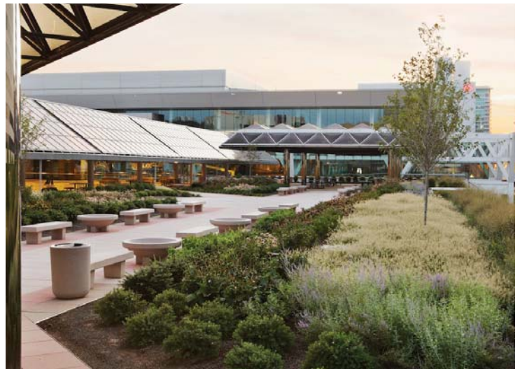
Baltimore Convention Center Green Roof
