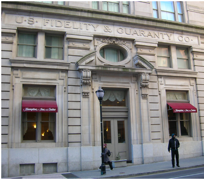
The awnings and signage respect the existing features.
