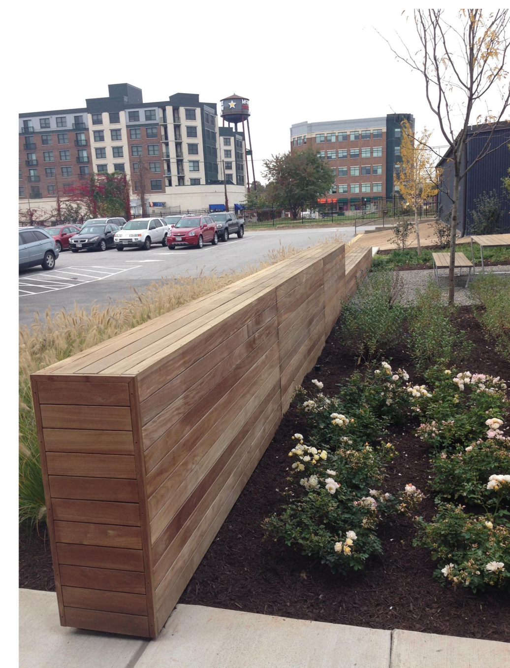
IPE-CLAD CONCRETE WALLS
