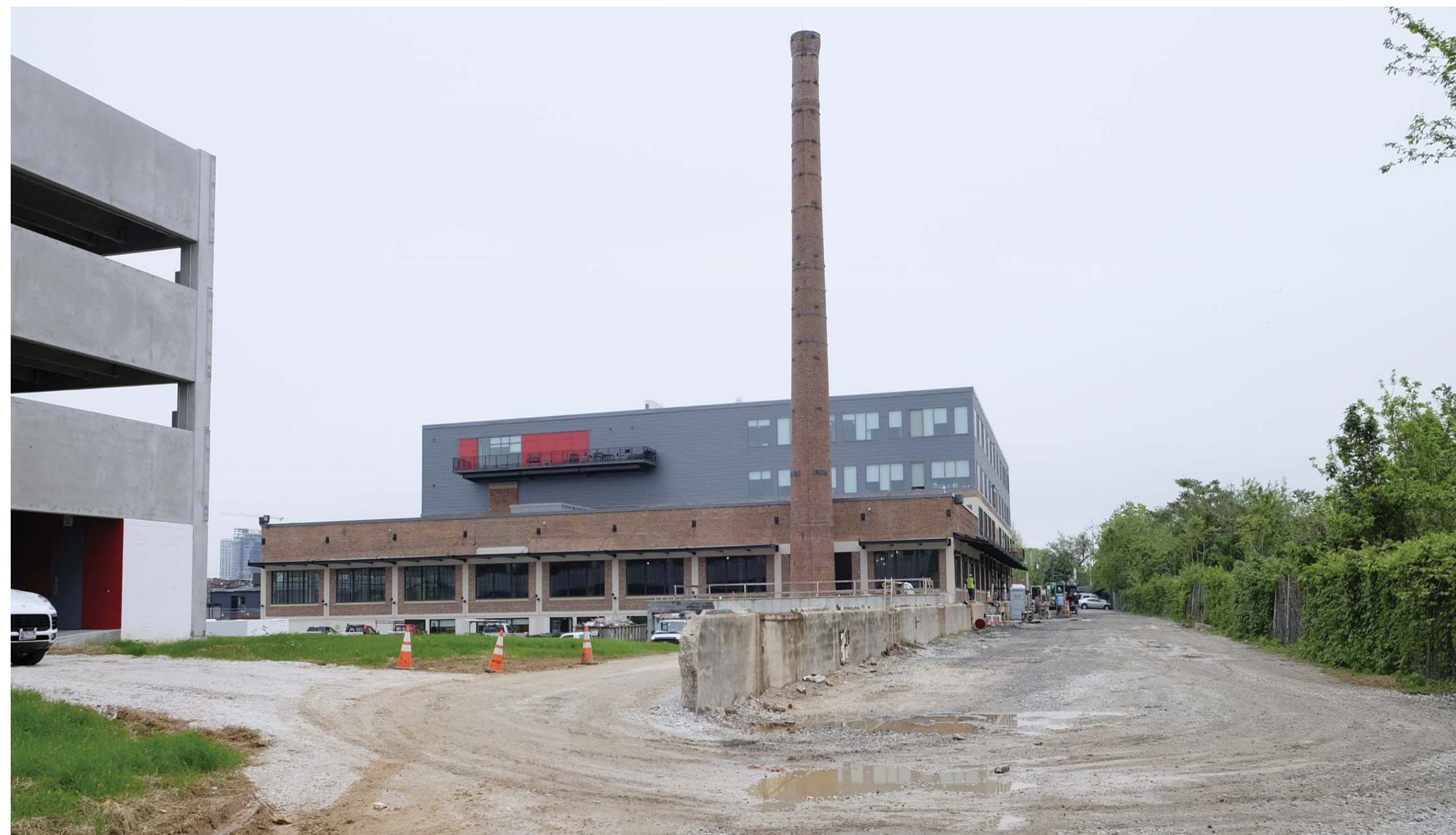
5. VIEW FROM EXISTING PARKING LOT INTO SITE AFTER DEMOLITION
