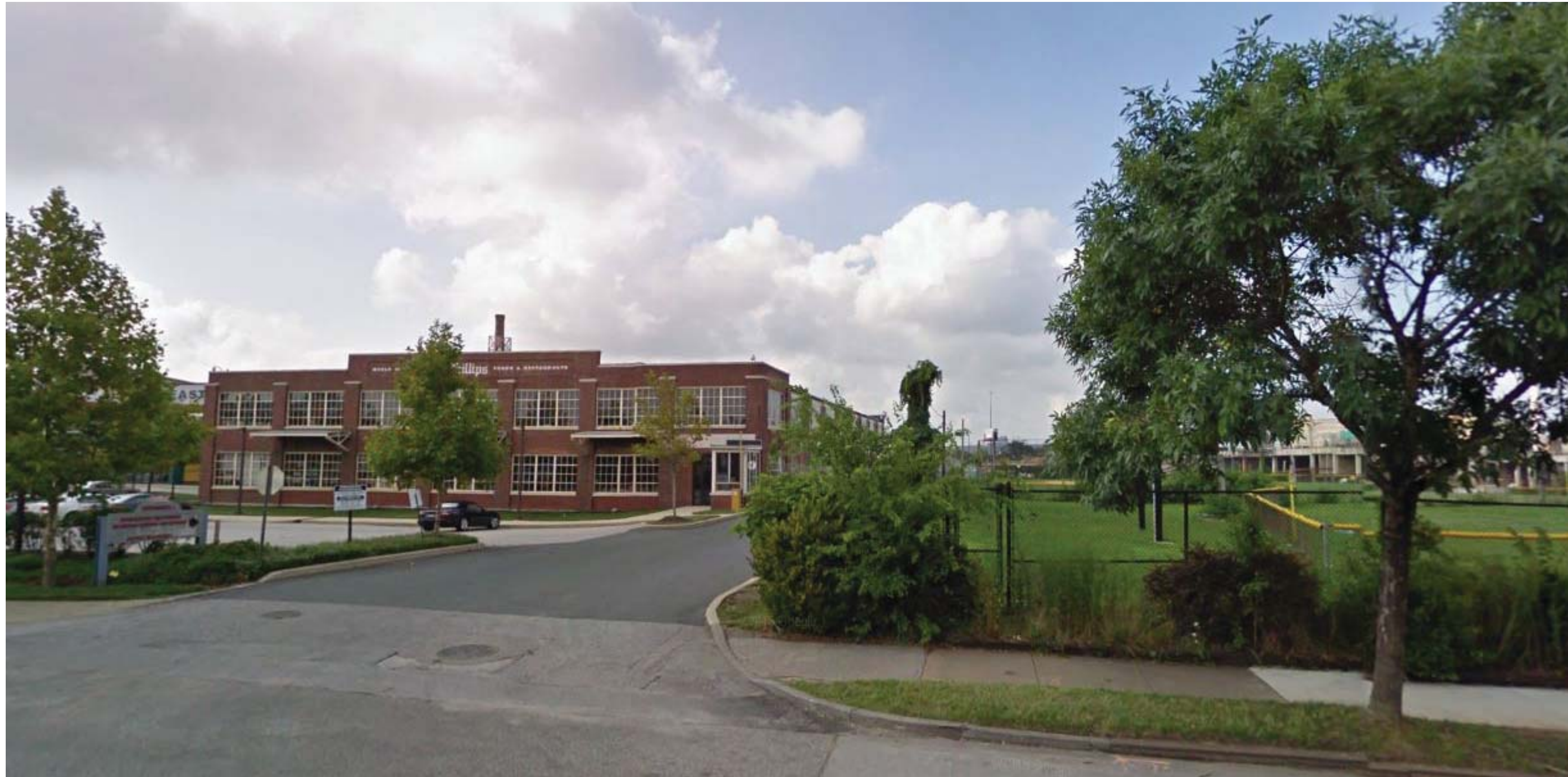
1. VIEW FROM E FORT STREET INTO EXISTING BUILDING
